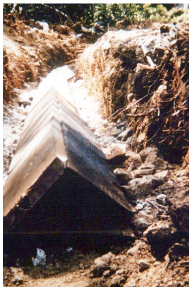
Photo 1. Early Vee Notch Leaching Trench Under Construction
